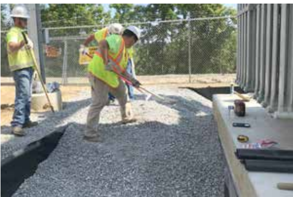
Covering liner with clean, washed stone
