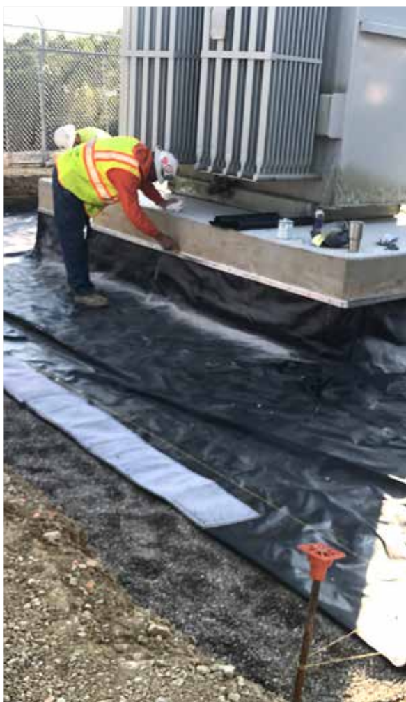
Connecting liner to concrete pad
