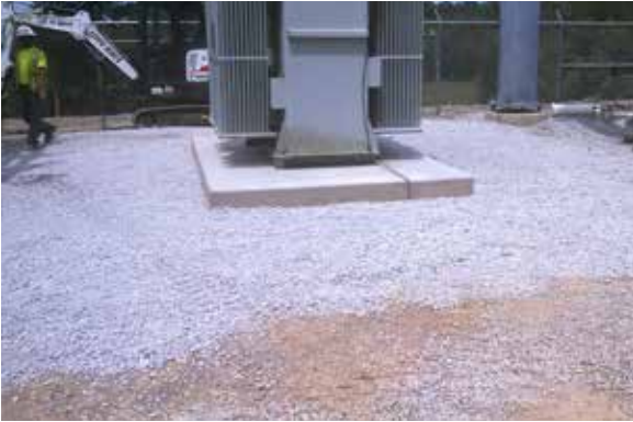
Completed to-grade installation
