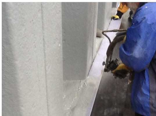
Steel sheeting application.
