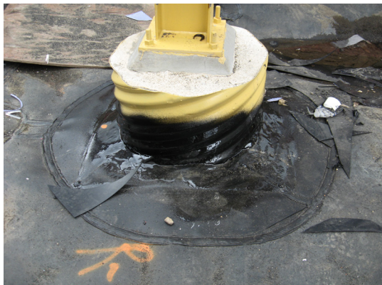
Pipe support application.
