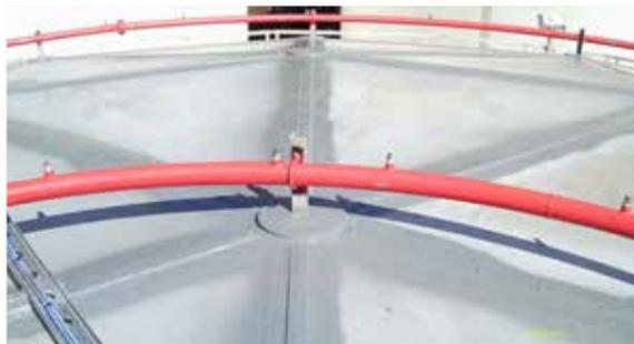
Gaps between panels completely sealed
