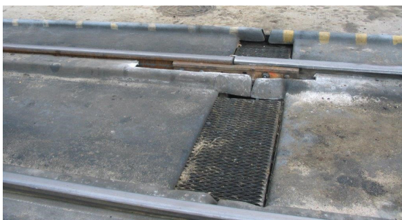
Rail pan prior to repair
