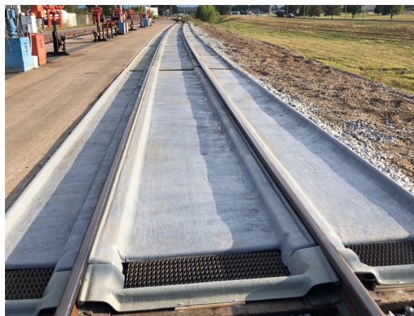
Rail pan after Justrite's SC-3900 coating
