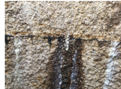
Grout injection at several places around the leak to ensure the water source is stopped. Leak 100% sealed and ready to be coated with SC-3900 Lining System.
