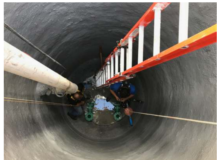
Grout injection at several places around the leak to ensure the water source is stopped. Leak 100% sealed and ready to be coated with SC-3900 Lining System.
