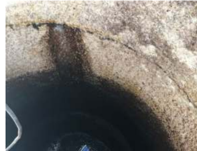
Active leak in a liftstation joint. Crews start to drill into the area around the joint to prepare for grout injection.
