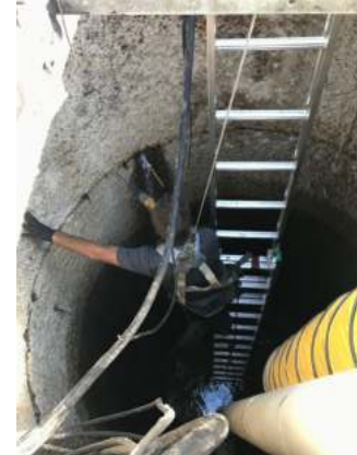
Active leak in a liftstation joint. Crews start to drill into the area around the joint to prepare for grout injection.
