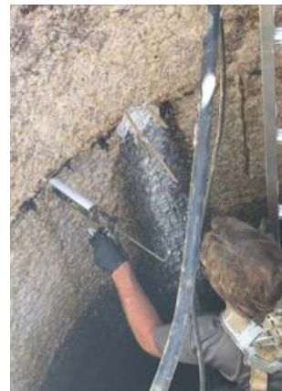
Grout injection at several places around the leak to ensure the water source is stopped. Leak 100% sealed and ready to be coated with SC-3900 Lining System.
