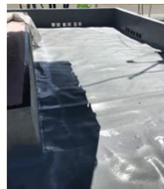
Pre-fabricated panels with field-applied SC-3900 seaming and connections allow for faster installations.
