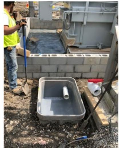
Use optional HFF passive drainage system to ensure SPCC compliance.
