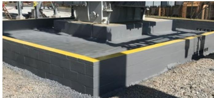
Containment size and shape can be designed to meet site geographical requirements. Identify your containment structure with safety yellow markings.
