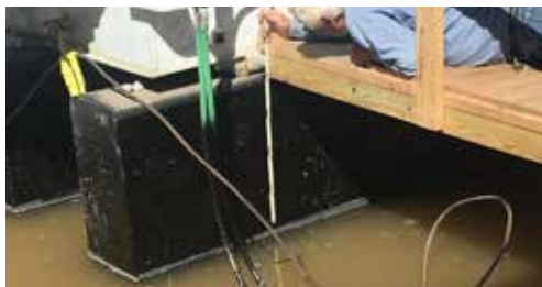
Performing hydrostatic pressure test
