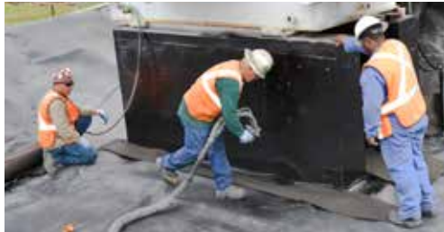
Sealing transformer pad with PolySeam.
