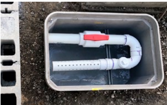
HFF provides passive drainage for containment wall system
