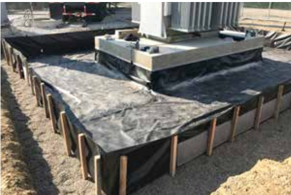
Liner installation around transformer
