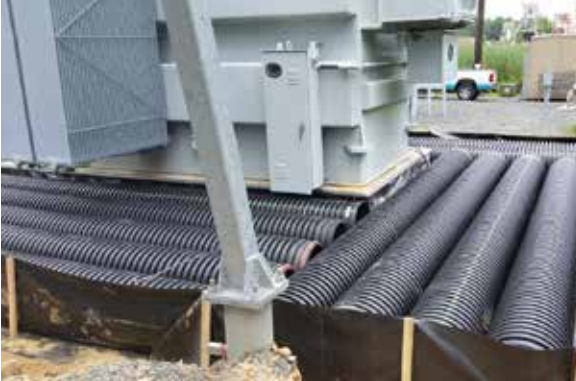
Increase void space with HDPE pipes
