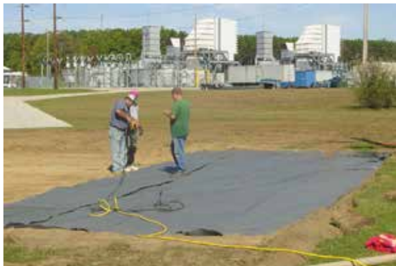
Land cleared and Agent-X is rolled out.
