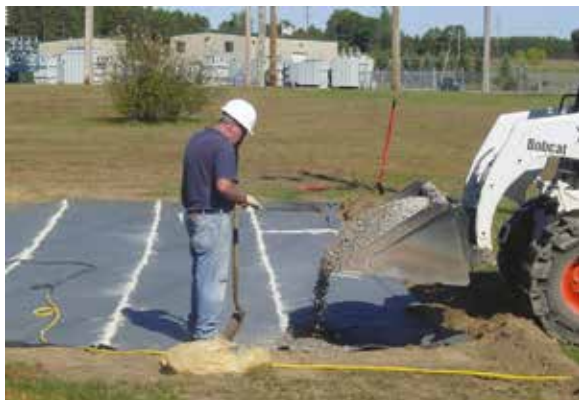
Bentonite clay placed over the seams. Gravel is then placed over the material.
