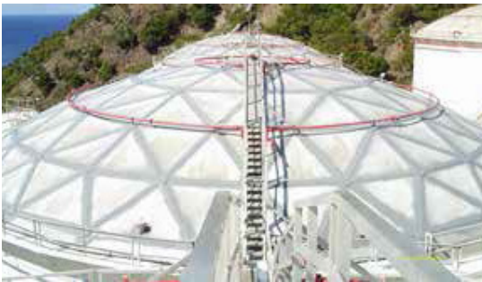
Geodome roofs sealed with SC-3900.
