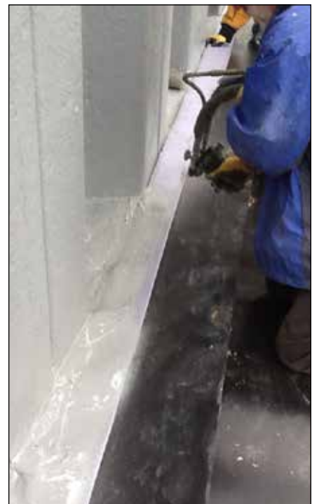
Steel sheeting application
