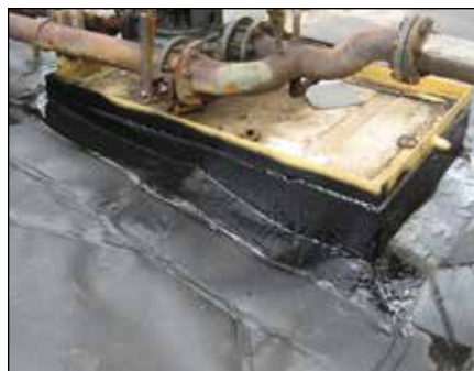
Pump pad application
