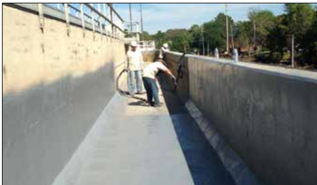
Spray technology repairs cracks and leaks.
