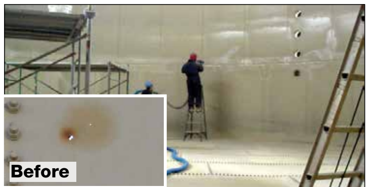
Holes in tank were repaired using our structural coating system.
