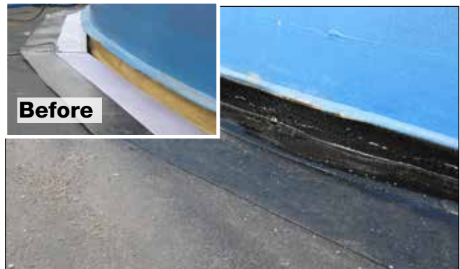
Double-bottom tank sealed with PolySeam® prevents water from going under the tank, no corrosion.
