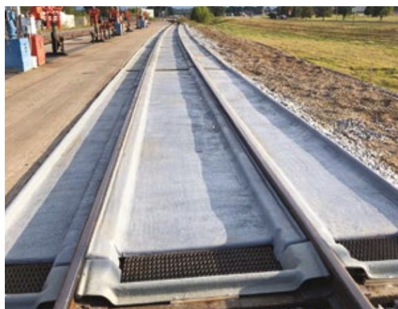
Rail pan after BCI's SC-3900 coating
