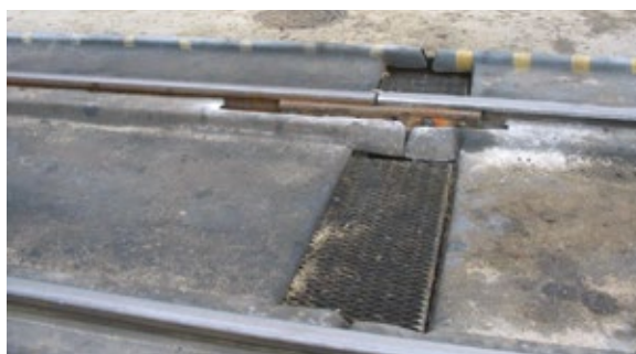
Rail pan prior to repair
