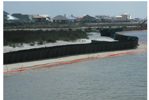
Sheen Boom deployed along north shoreline of Dauphin Island, Ala., after Deepwater Horizon Oil Spill (May 2010).
